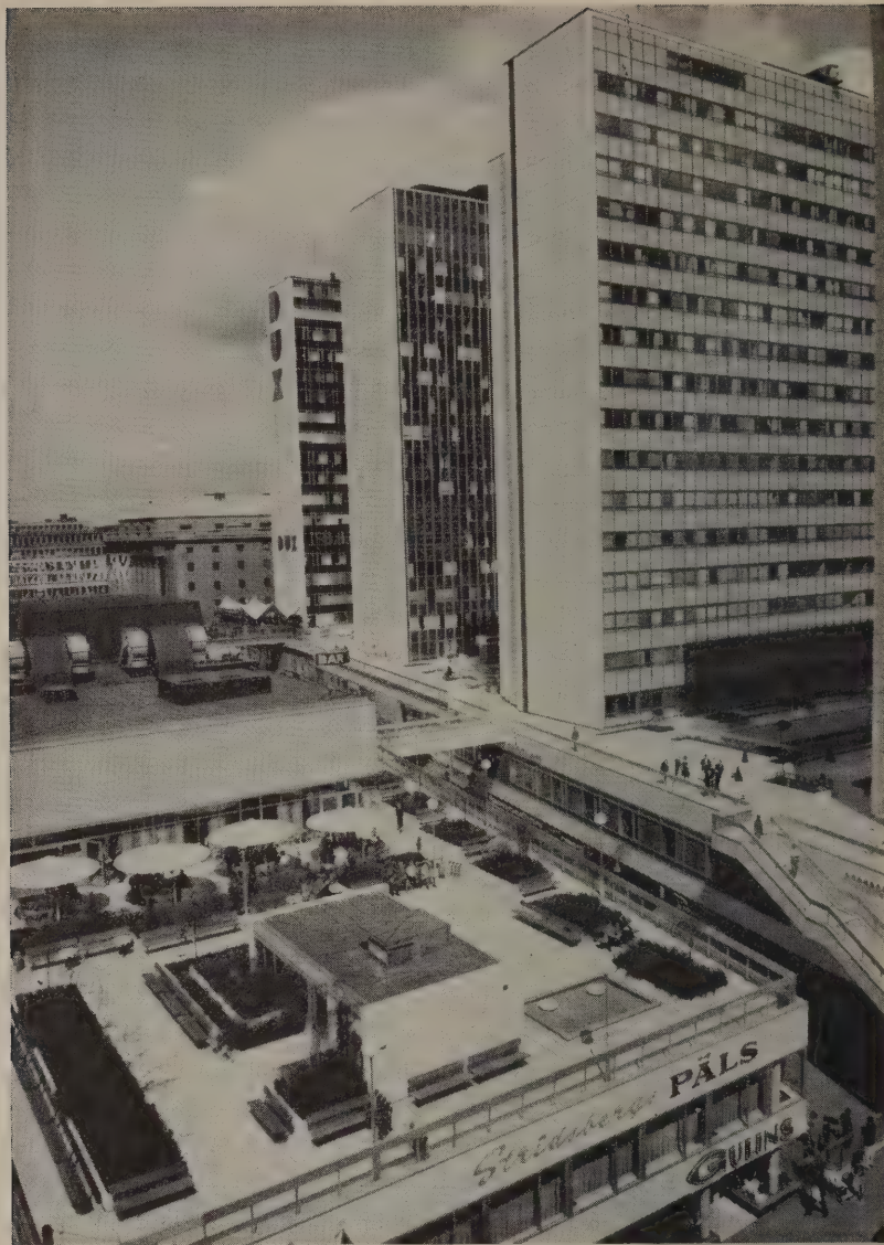
233 Stockholm. The multi-level reconstruction in the centre.
